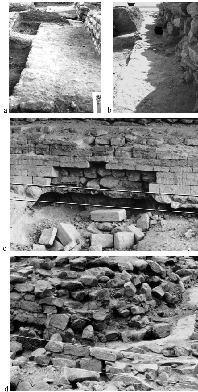
Fig. 7: Layer 3 foundation for outer facing at Sinki NW side (a), Seila east side (b) Hebenu north side (c) and Elephantine east side (d).
